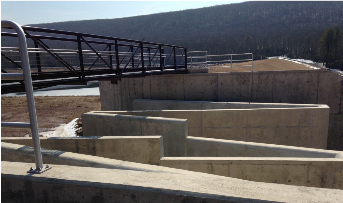
Fig. 1. Staged labyrinth weir at Upper Owl Creek Dam, Tamaqua, PA
