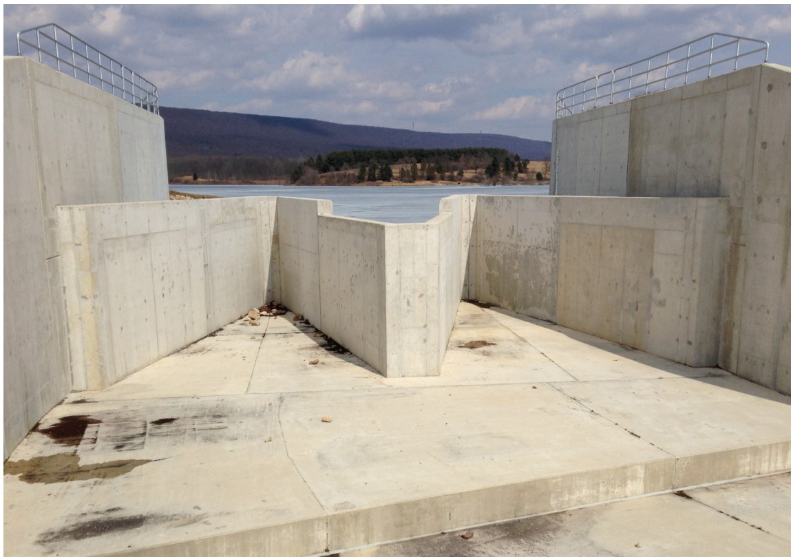
Fig. 2. Staged labyrinth weir at Leaser Lake Dam, Fogelsville, PA
