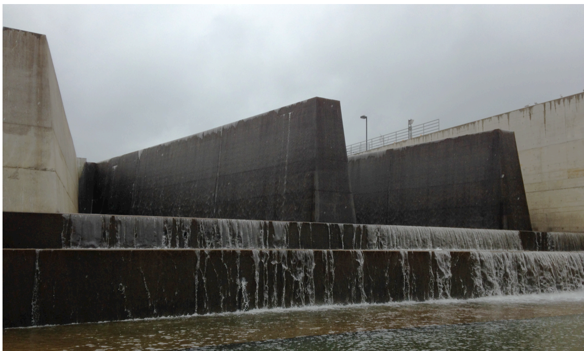
Fig. 3. Staged labyrinth weir at Lake Townsend Dam, Greensboro, NC
