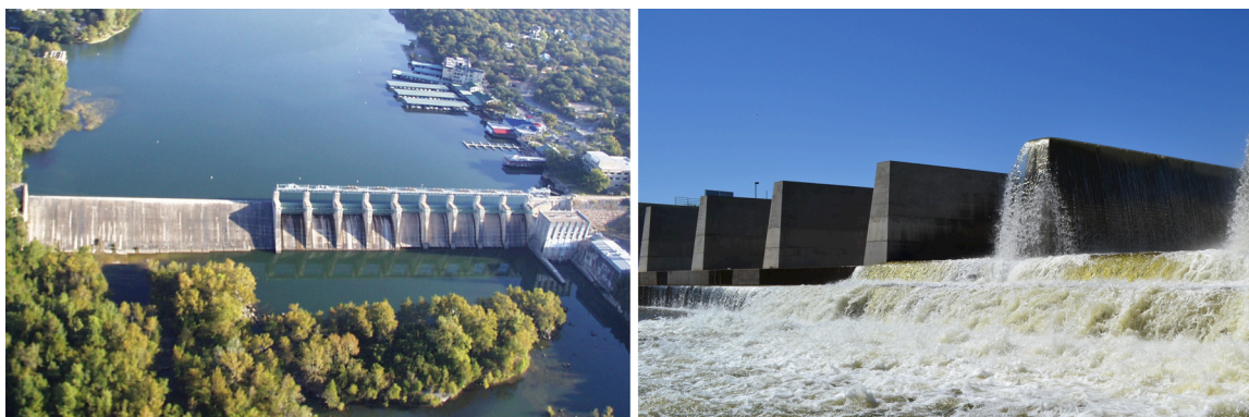
Fig. 21. Photos of staged ogee-crested weir (Tom Miller Dam, TX) and staged labyrinth weir (Lake Townsend, NC). Courtesy of: Michael Johnson and Brian Crookston
